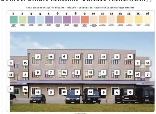
Fig 4: The External side of the Bollate prison
